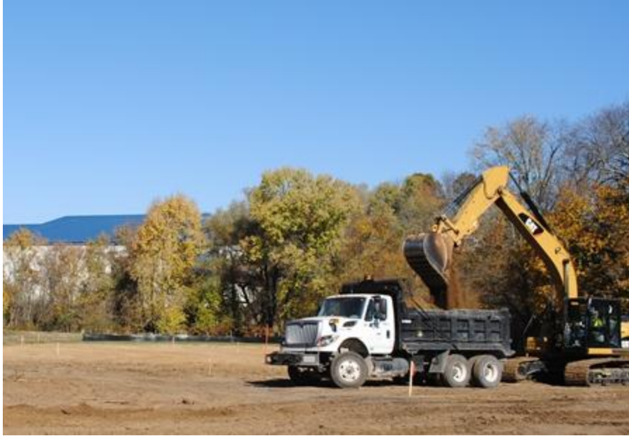
Town Crews leveling the multi-purpose field.
